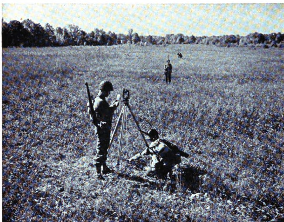
Figure 27. Survey crew establishing preliminary center line.
